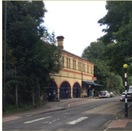
Maidenhead Railway Station access off Shoppenhangers Road
