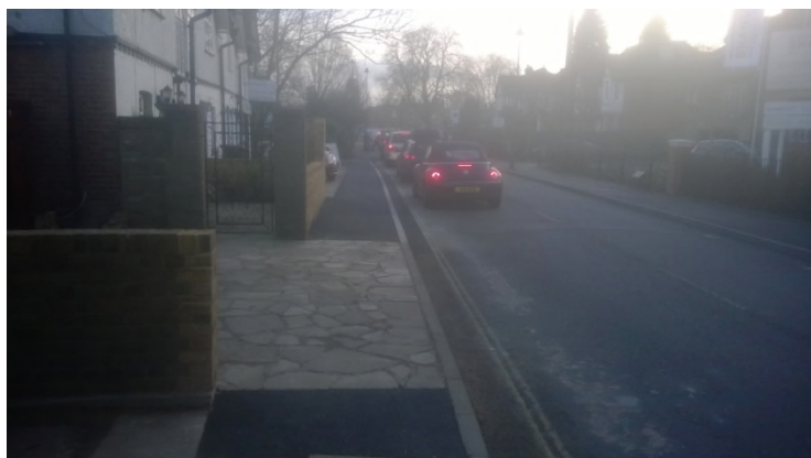
Thames Path link after with pavement created
