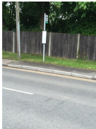
Bus stop kerbs
