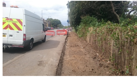
A308 Maidenhead Rd cycleway under construction
