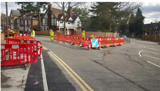
Osborne Rd/Francis Rd under construction
