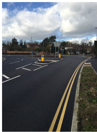
Completed Stafferton Way/Oldfield Road junction
