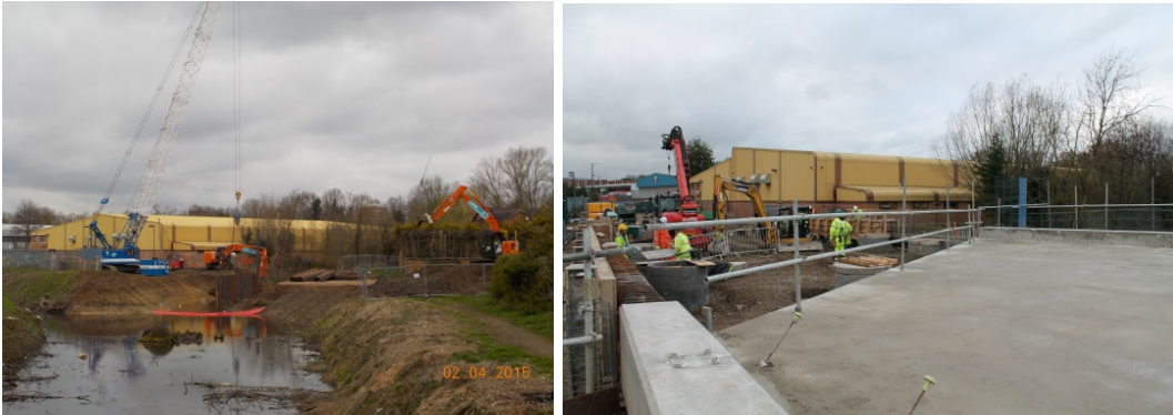
Stafferton Way under construction
