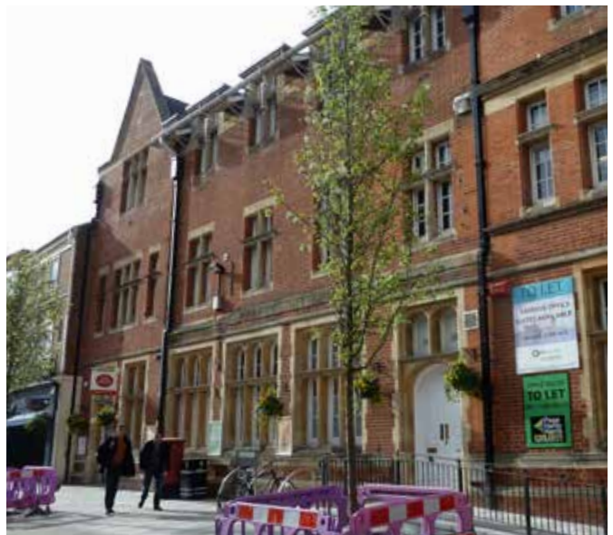
The Post Office (building of local significance)
